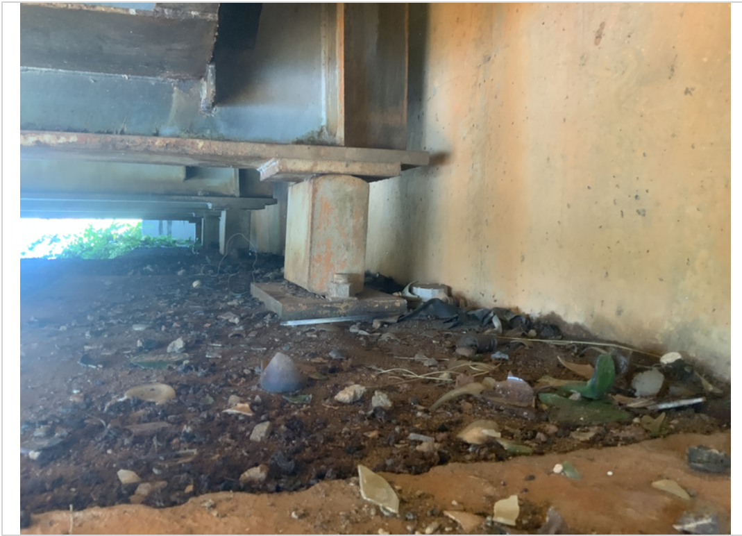
Abutment 4, rocker bearings. 2021
