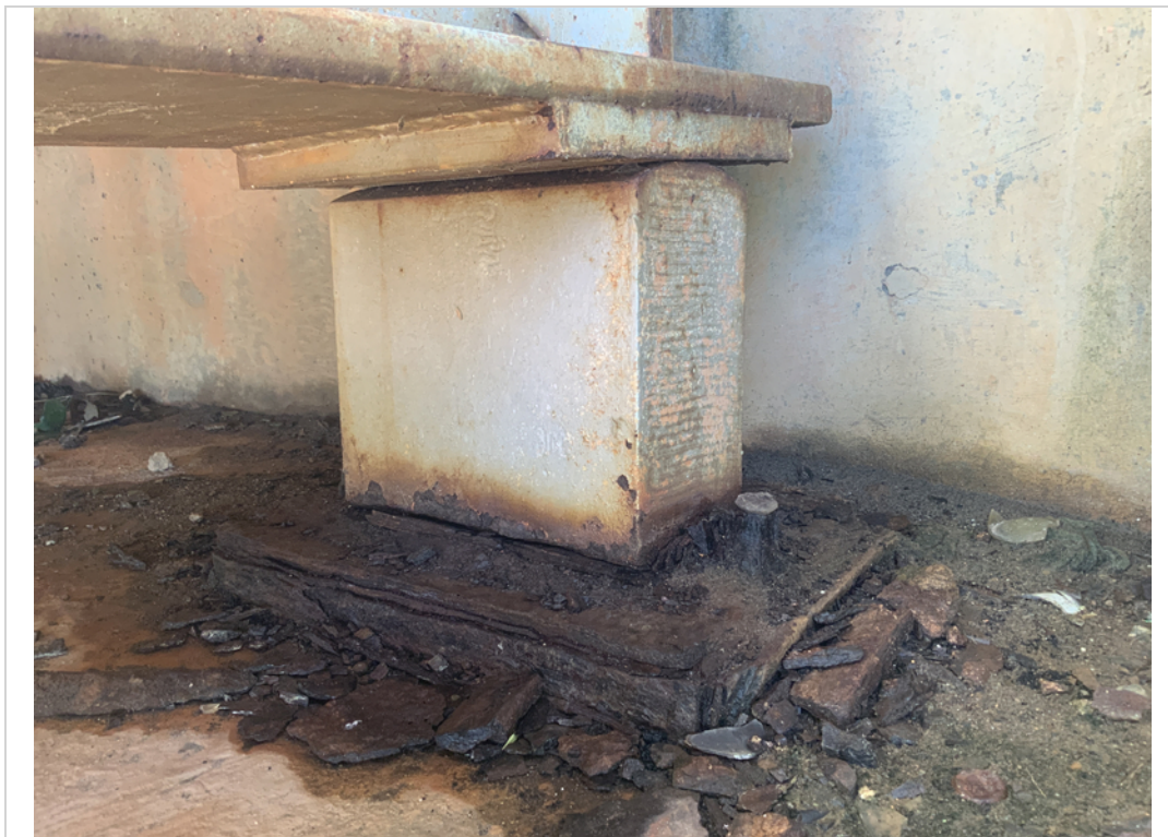
Abutment 4, bearing 5 corrosion. 2021
