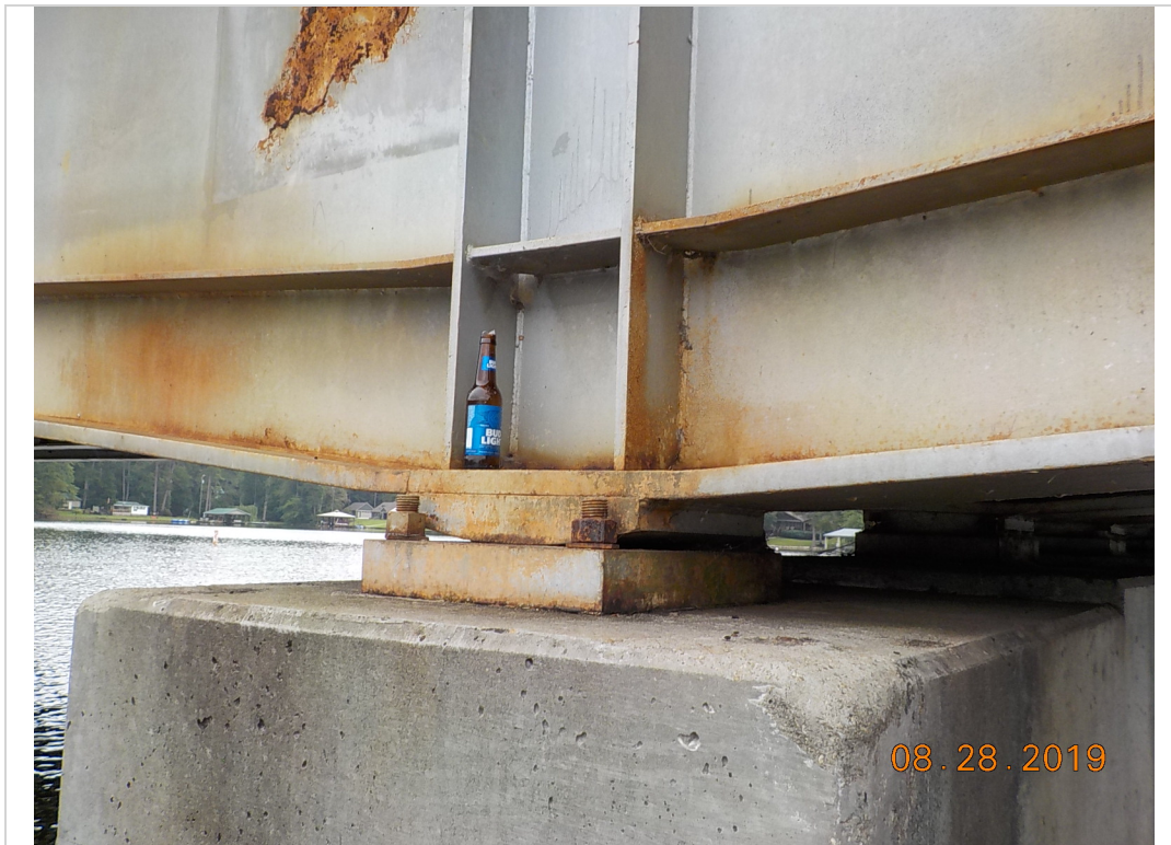
Bearing assembly at bent 2
