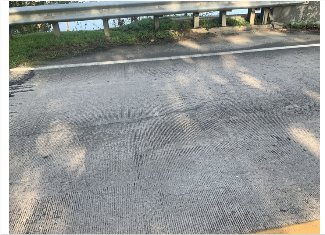
Rear approach slab longitudinal cracking. 2023
