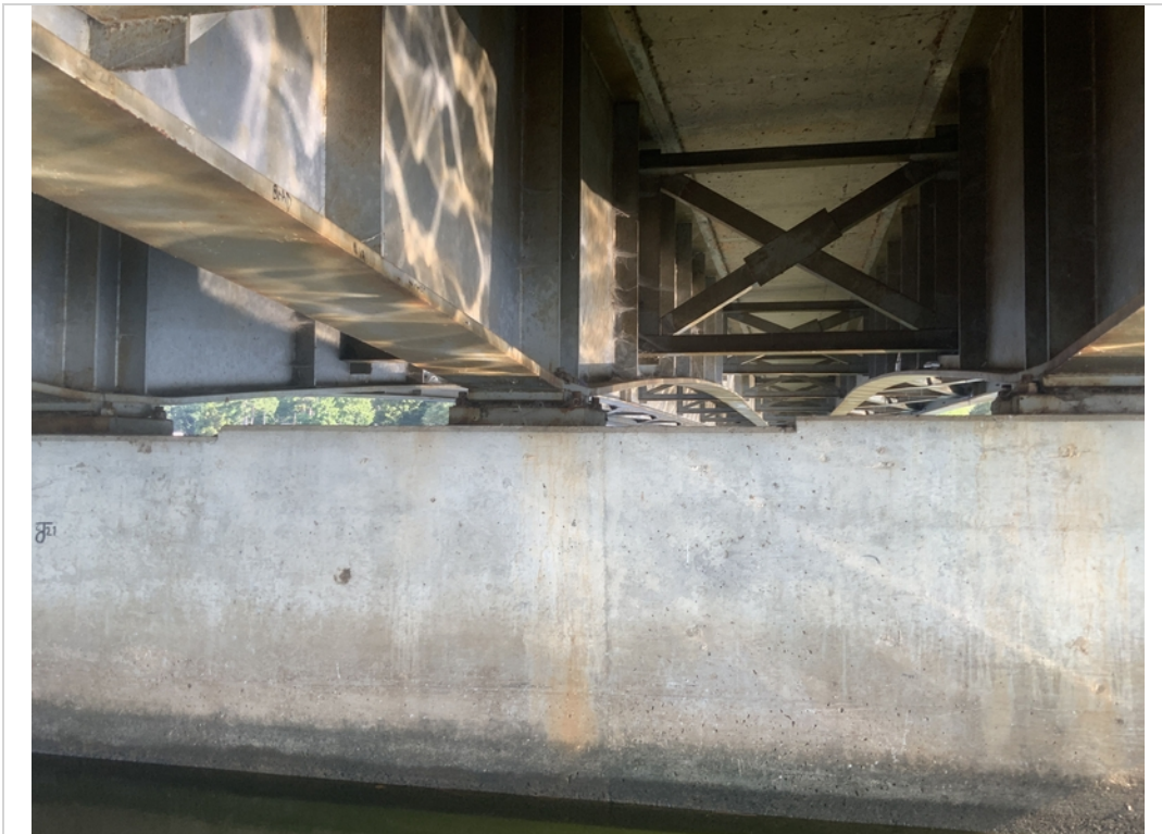
Bent 2 bearings. 2023
