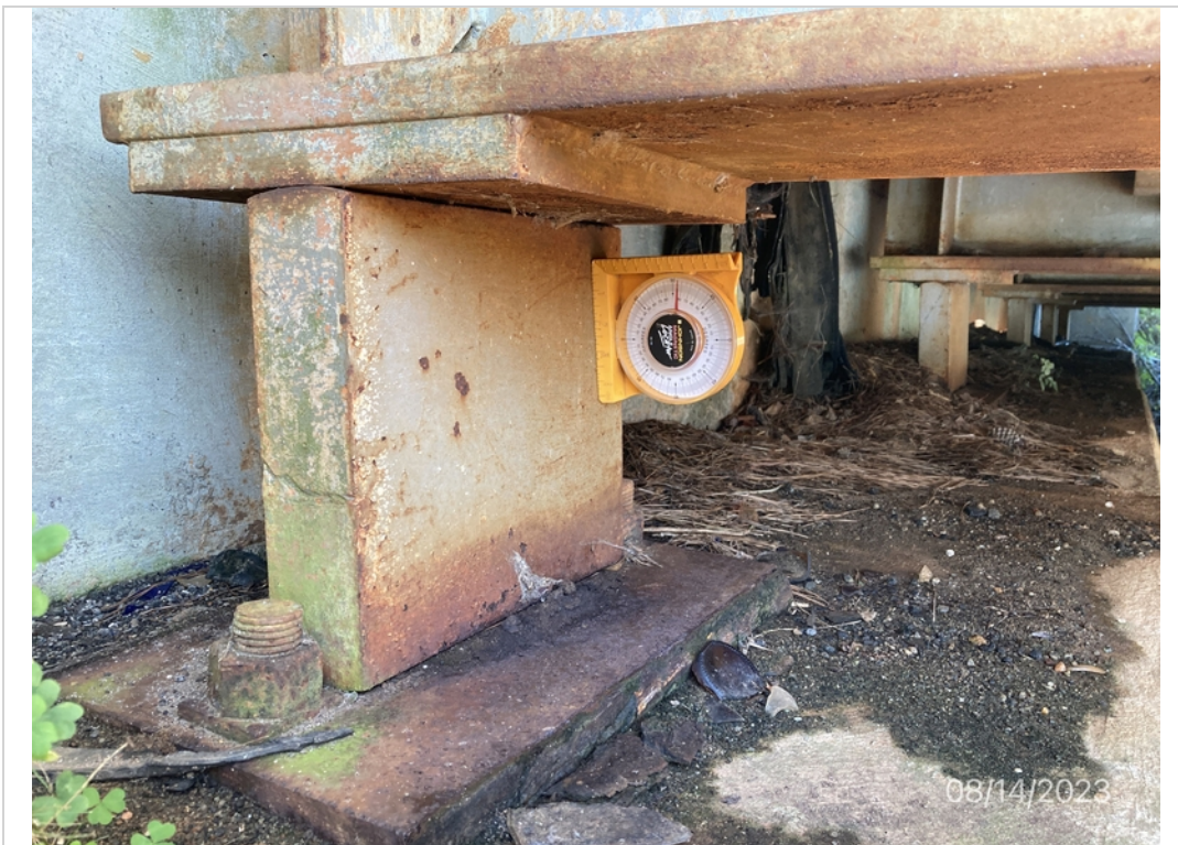
Abutment 1 rocker bearing tilt. 2023
