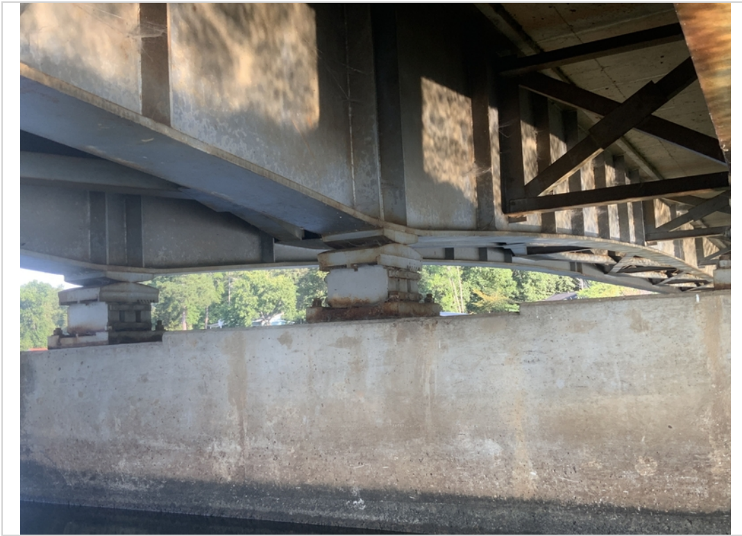
Bent 3 rocker bearings. 2023
