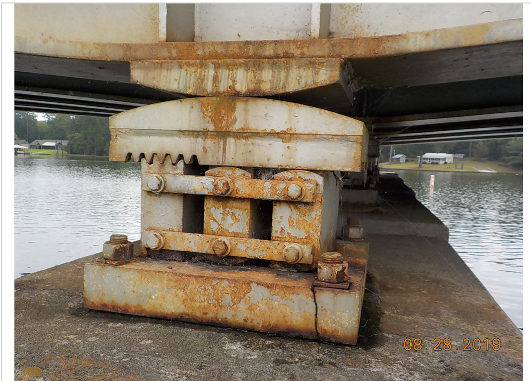
Bearing assembly at bent 3
